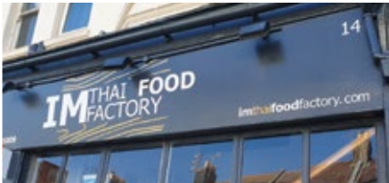
Vinyl applied to existing fascia
