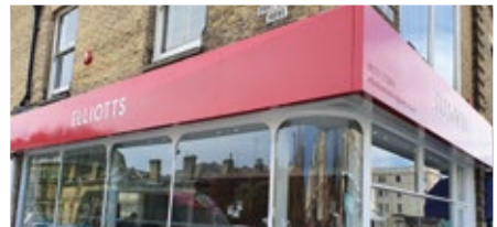
Aluminium sign tray fret cut with internal illumination
